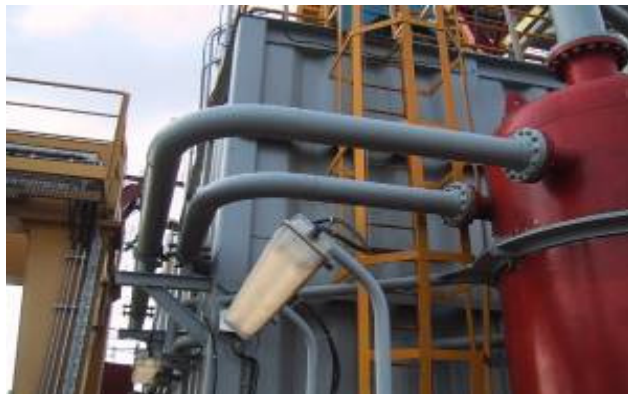
Figure 1 – Short-sweep ells downstream of choke
